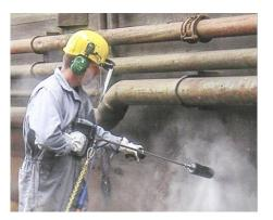
**1st Gear**Low pump power for manual blasting gun work
