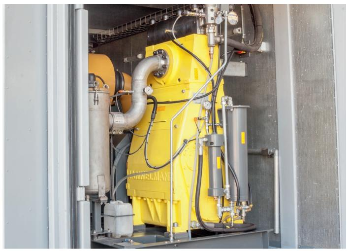
Stationary diesel unit in a soundproof container
